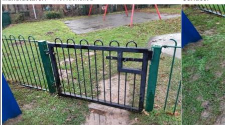
**Finding:** The area under the gate has eroded leaving uneven areas, or the concrete foundations exposed, resulting in trip hazards at the entrance/exit to the playground
