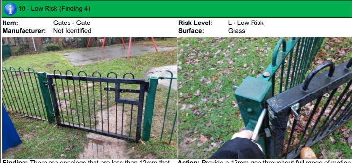
Finding: There are openings that are less than 12mm that could trap or crush fingers
