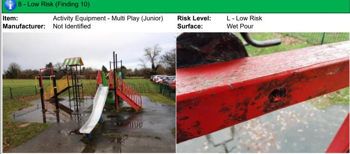
Finding: The fixings have corroded excessively
