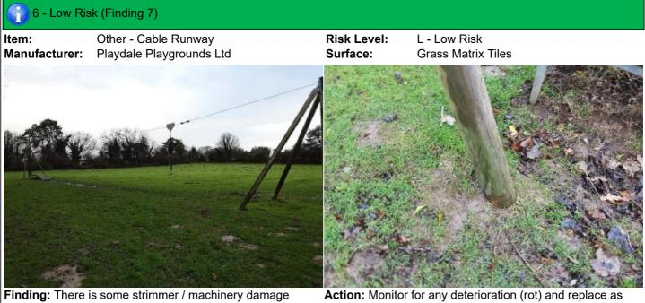
apparent on the posts, this can penetrate the preservative applied to the timber and accelerate the rotting process
