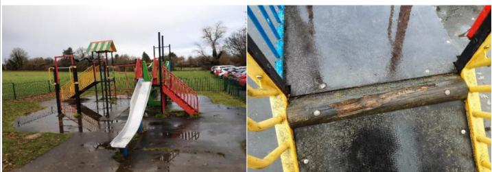
Finding: There are areas or parts of the timber on the ramp Action: Replace all affected timbers treads that have rotted
