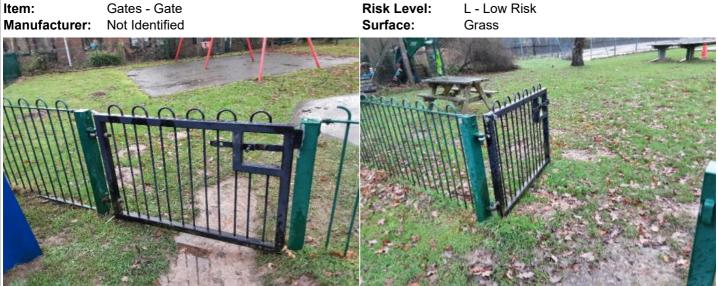
Finding: The self closing mechanism is missing from one of Action: Replace the gates
