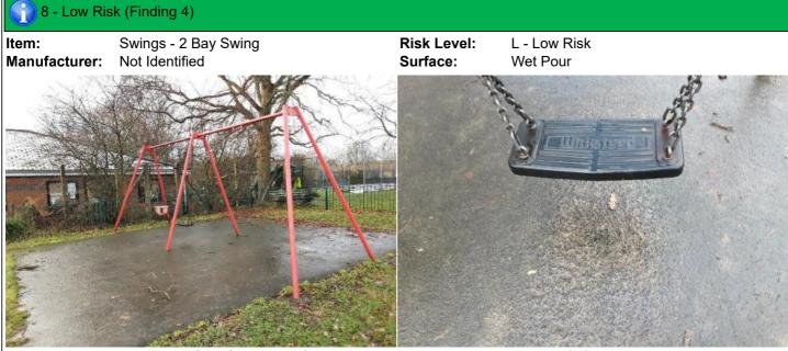
**Finding:** The seat clearance from finished surface level to the underside of the seat is too low and does not meet the requirements of BS EN 1176 Part 2 (350mm minimum clearance required)
