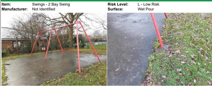
**Finding:** The surface has eroded and the foundations are exposed
