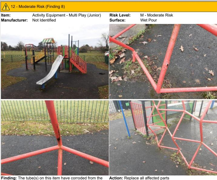
**Finding:** The tube(s) on this item have corroded from the inside and split the steel
