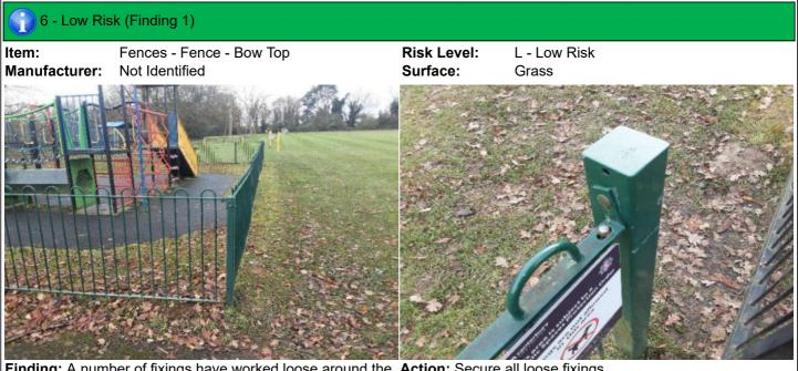
**Finding:** A number of fixings have worked loose around the **Action:** Secure all loose fixings fencing
