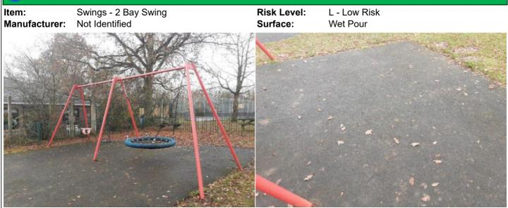
Finding: The safety surface around the area is beginning to Action: Monitor for any further deterioration and repair as required
