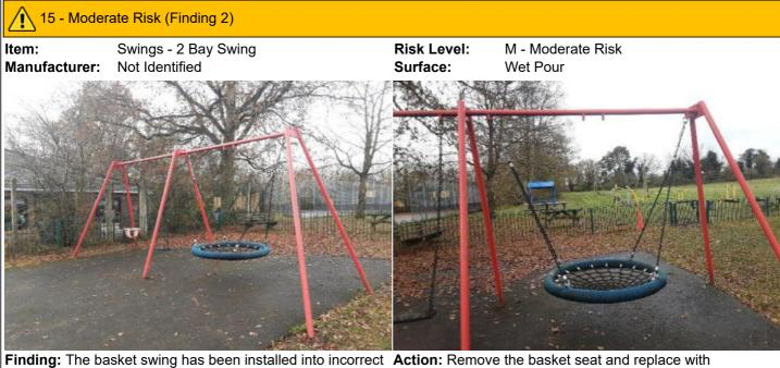
**Finding:** The basket swing has been installed into incorrect frame design and is wearing the connecting points excessively
