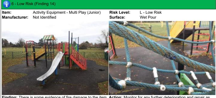
Finding: There is some evidence of fire damage to the item Action: Monitor for any further deterioration and repair as required
